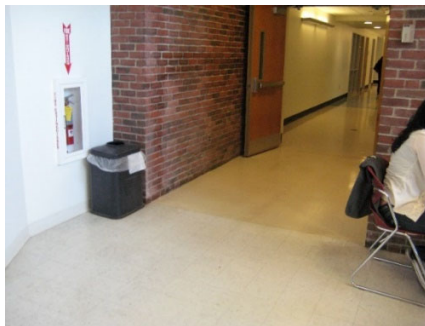
Figure 3: Example of flooring material that is known ACM located in the Iddles wing of Parsons Hall
