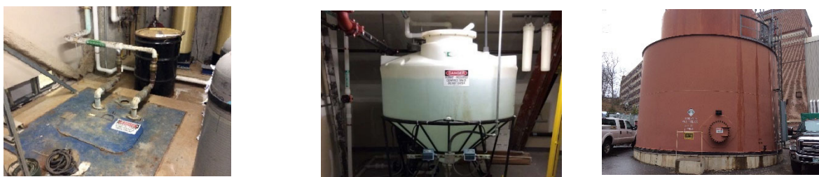
Figure 7: Equipment identified as a Permit Required Confined Spaces
